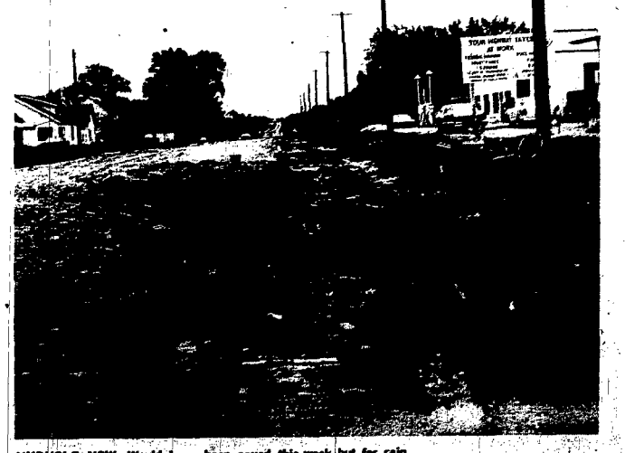
MUDHOLE NOW. Would have been paved this week but for rain.
